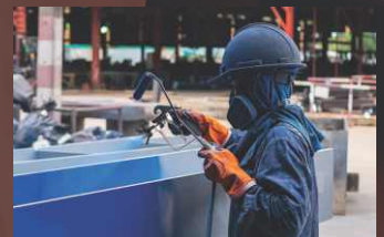
PEB & industrial structural fabrication
