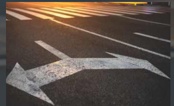
Road marking & curb coatings
