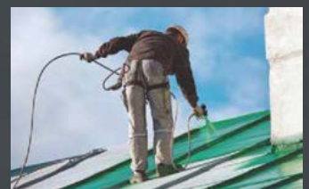
Flooring and roof coatings
