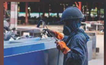
PEB & industrial structural fabrication
