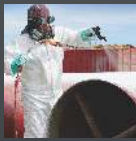
Pipe & other protective coating
