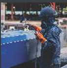
PEB & industrial structural fabrication
