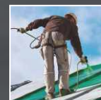
Flooring and roof coatings
