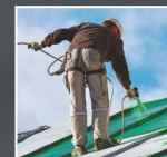
Flooring and roof coatings
